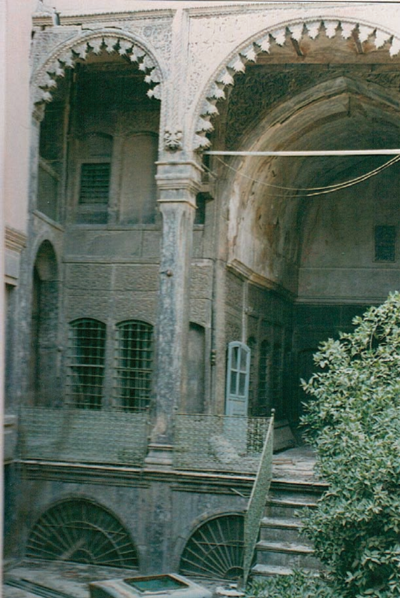
Fig (4) Arch of the aiwan in the traditional house of Mosul city
